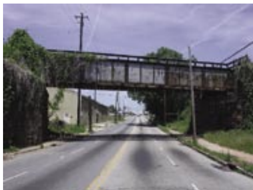
Figure 6.22 Pryor Street Before
