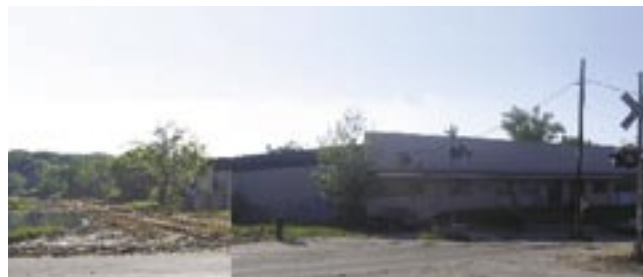
Figure 6.27 Boulevard Crossing Before
